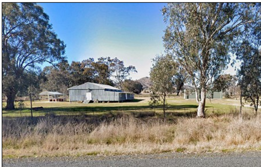
A photo of the Mullengandra Hall from Bowna Road, the old Hume Highway – see page 3
