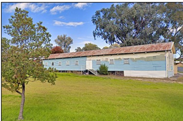
West Albury Community Hall before a recent restoration *
