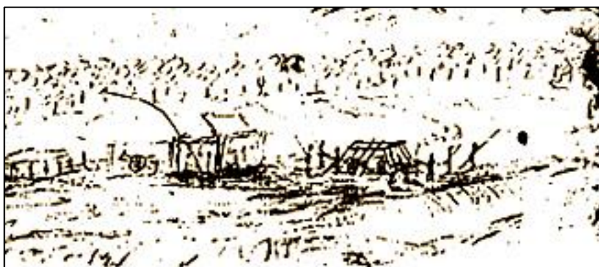
Robinson sketched Stuckey's substantial fortress. The small slab hut (3.6 x 2.4m) was capable of protecting eight people with loopholes facing in all directions.
