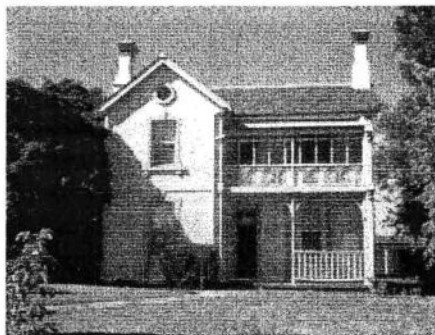
Photo 1: Station Master's Residence, Young St/ Railway Place.
