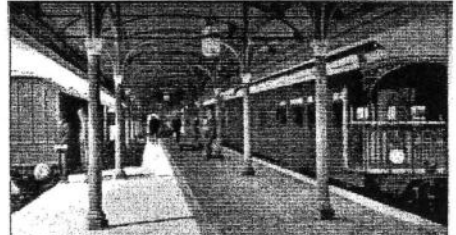
Photo 14: Albury Railway Platform.
