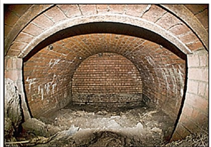
Rapid Survey of a Subterranean Structure at the Albury Pioneer Cemetery
