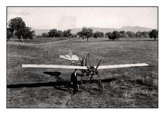
On Tuesday the experiment was repeated in the presence of a Banner representative and the machine took to the air gracefully. The trial, however, was interrupted by a mechanical de-fect, but the test demonstrated the capacity of the monoplane to take to the air after a ground run of about 200 yards. The inventors, who deserve to be rewarded for their patience and industry, intend exhibiting their machine at the coming Albury Show.
