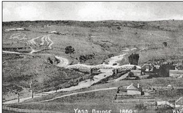
The first bridge over the river at Yass, 1860
