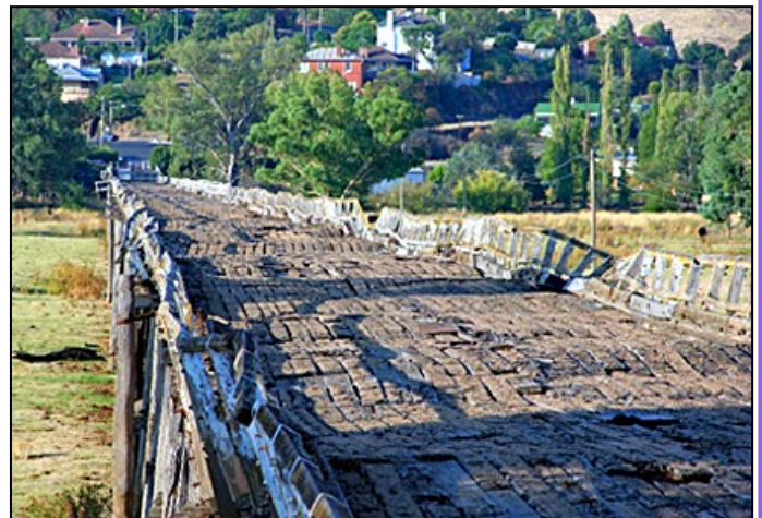
The old bridge at Gundagai had to be demolished due to its deterioration.
