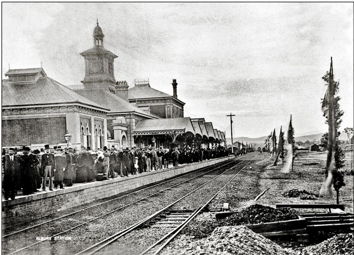
February 1881, the scene at the not yet complete Albury Railway Station as the train approaches carrying dignitaries from Sydney to celebrate the completion of the Great Southern Line
