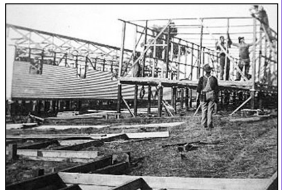
Construction at Bonegilla
