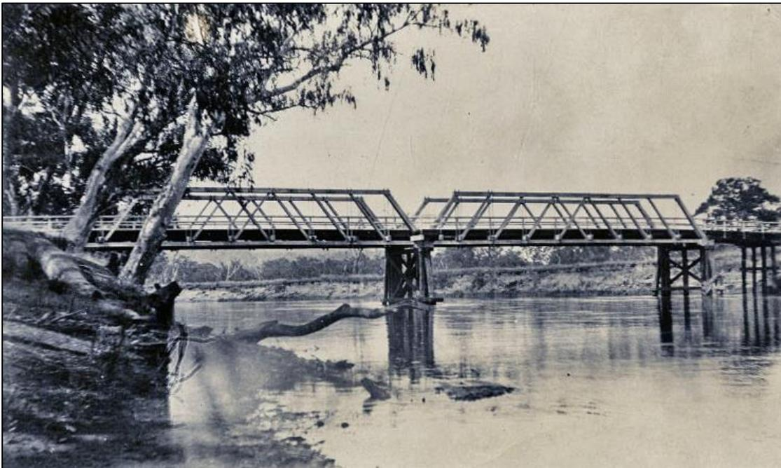
The bridge was built to a new design of Percy Allan, a young engineer in the NSW Public Works Department. It had two 90ft (about 28m) timber truss spans with two 30ft approach spans. The contract price was £1751, half borne by each of NSW and Victoria.
