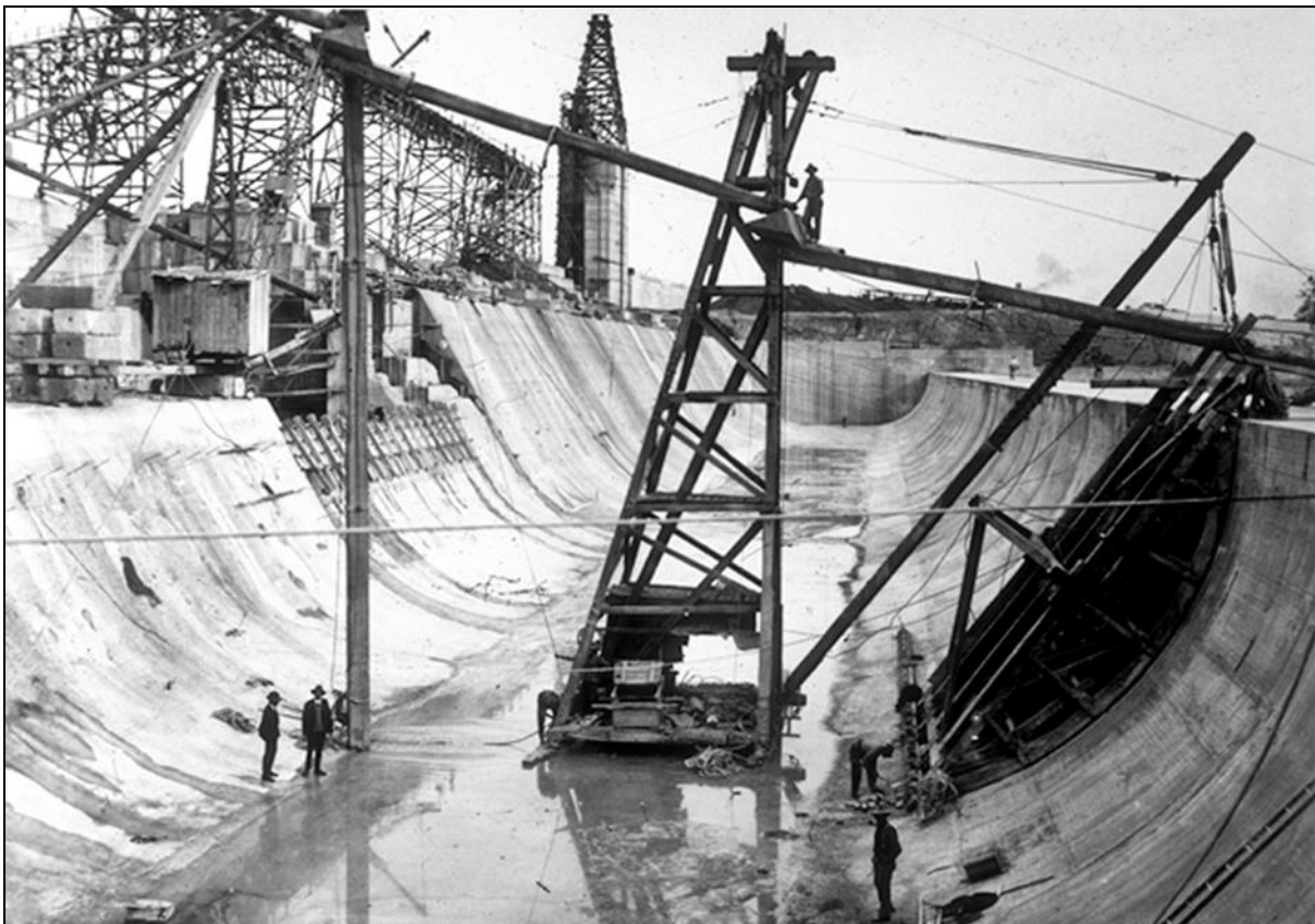
A dry dissipator trough and wall is not an everyday sight.
