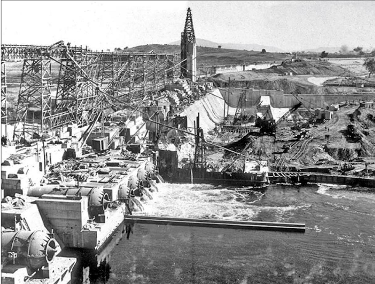
The four regulating valves are partly open while concrete is being delivered via four concrete chutes.
