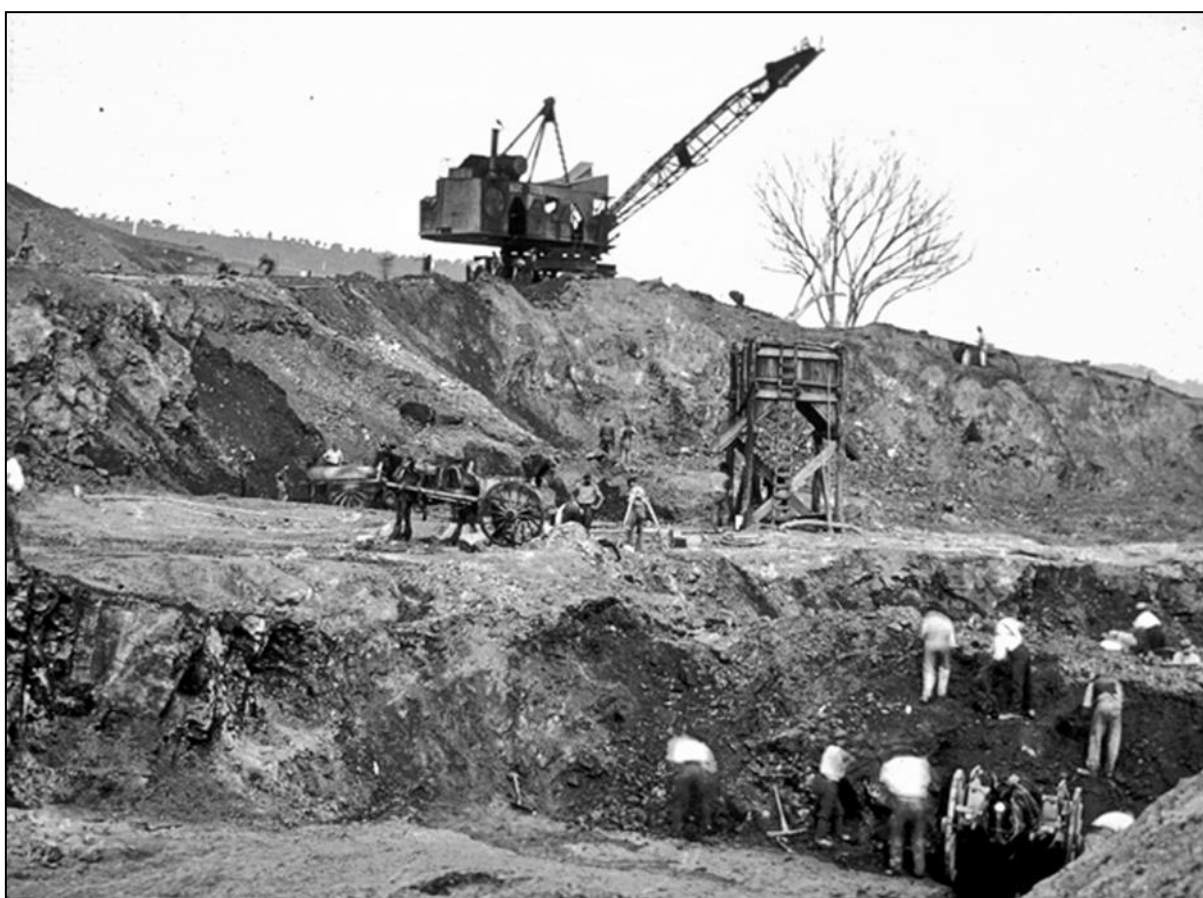
The Bucyrus steam shovel at work on the spillway site.
