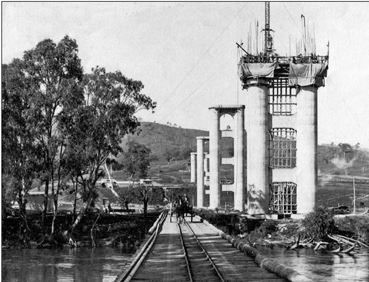
Four pylons on the Victorian side under construction c1928 showing the temporary bridge over the river.
