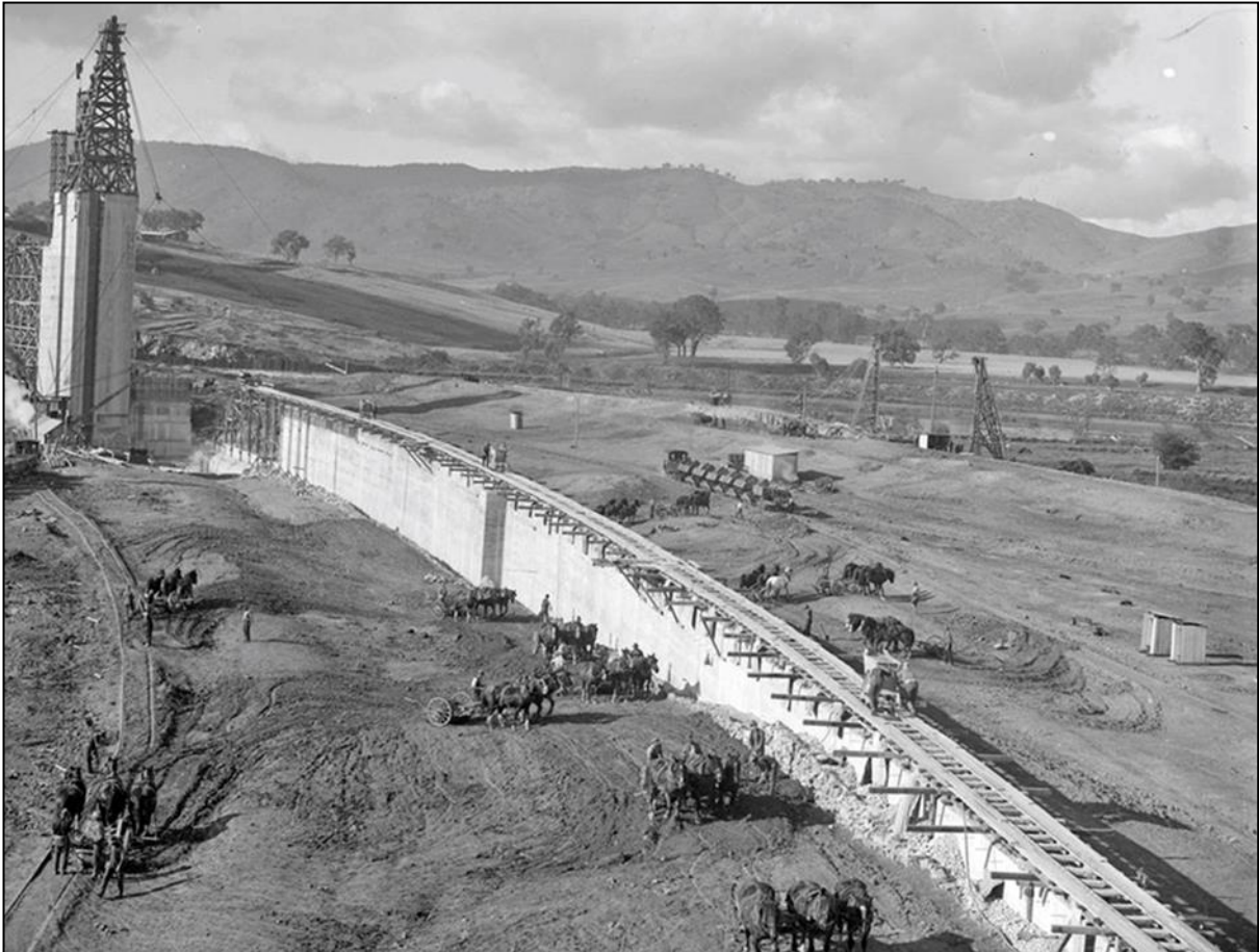
The Victorian core wall in 1930. The concrete wall eventually reached the height of the concrete tower on the left-hand side and 'keyed into' the dark slot. Bethanga Gap at top right.
