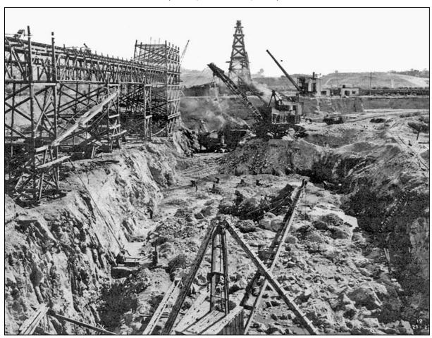
Looking towards the Victorian side – excavation for the foundation of the spillway and scene of the fatal explosion.
