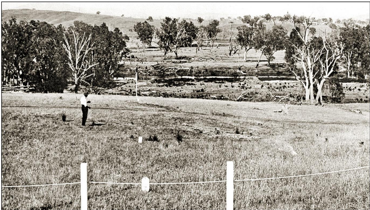
SURVEYING THE SITE: A surveyor working at the future site of the Hume Dam before construction commenced in 1919.
