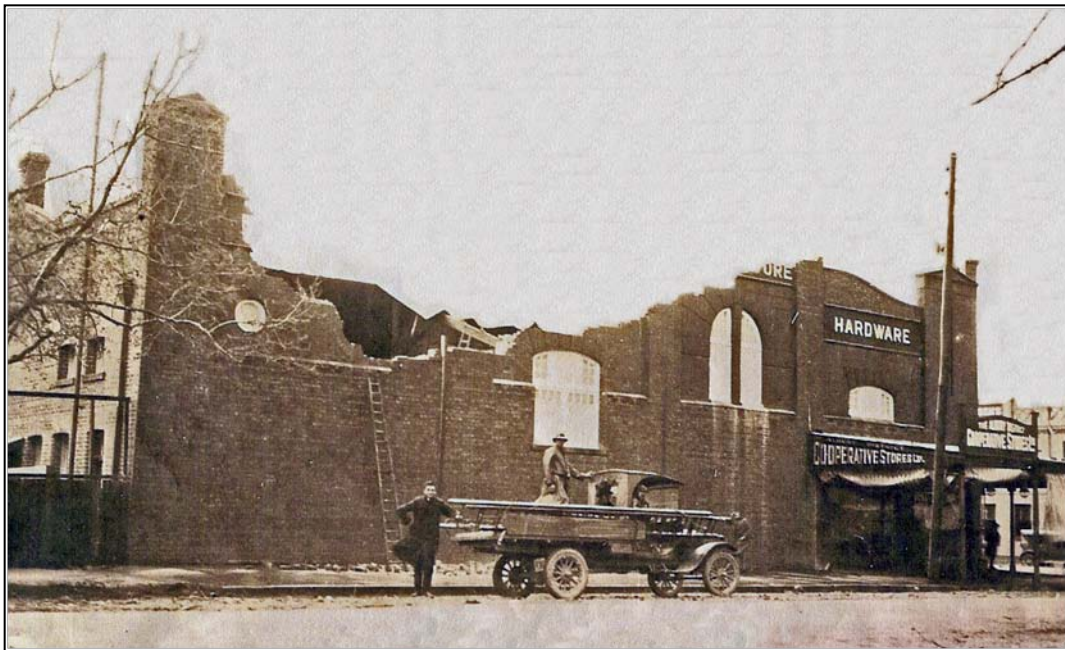
Damage to Reis' Model Store – Sodens Hotel far right
