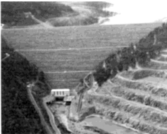
Dartmouth Dam showing the power station at the base of the dam and the stepped cascade below the spillway. (Photo Goulburn-Murray web site)
