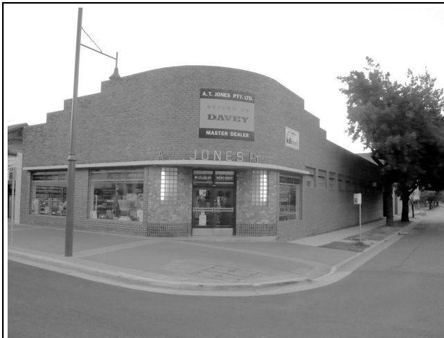
A T Jones building on the Corner of Kiewa & Stanley Streets 2008. The building extends across a resumed lane and two house blocks in Stanley Street. Bricks from the demolished houses were used to line a large cellar in which huge stocks of polythene pipe are stored.
