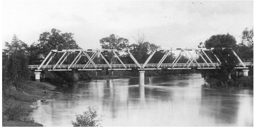
The second Union Bridge over the Murray River at Albury 'opened' by Frank Shepard on 31 December 1898 while working at the Brewery adjacent to the northern approach to the bridge. This bridge was constructed of timber and iron using the Howe truss design that had been adopted for road bridges in NSW in 1892. This bridge remained in use till 1961 when the current pre-stressed concrete bridge was opened.
