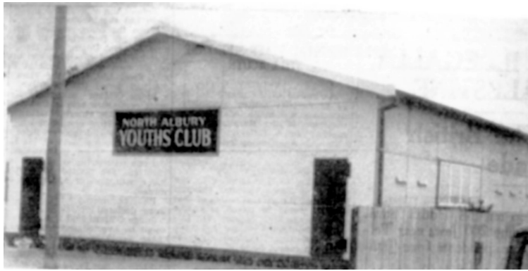
North Albury Youth Club Hall , formerly Red Shield Hut at Bandiana Army Camp, relocated to Buckingham Street 1946.
