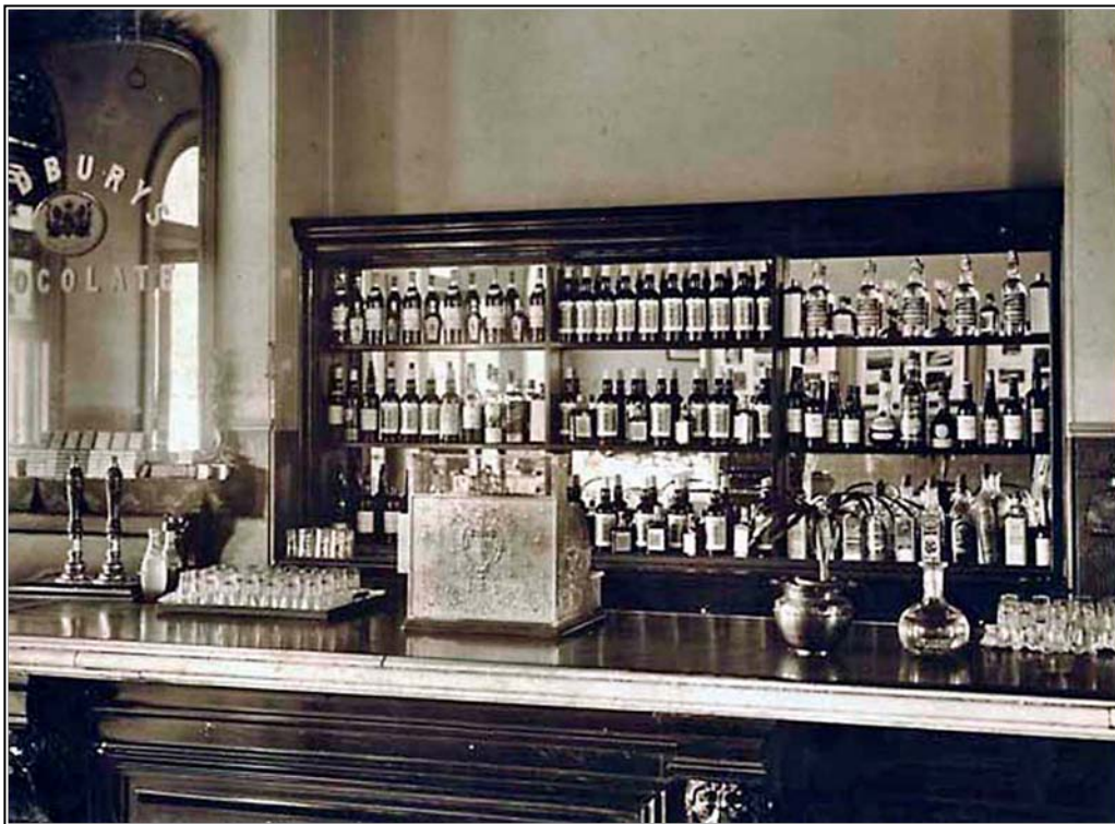
The well stocked bar area at Albury railway refreshment rooms (State Records NSW)
