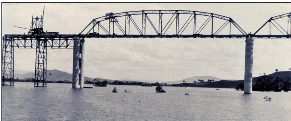
A rare picture of workmen perched in a cradle while riveting a steel span of the Bethanga Bridge in 1929. A "creeping crane" prepares for the next span.
