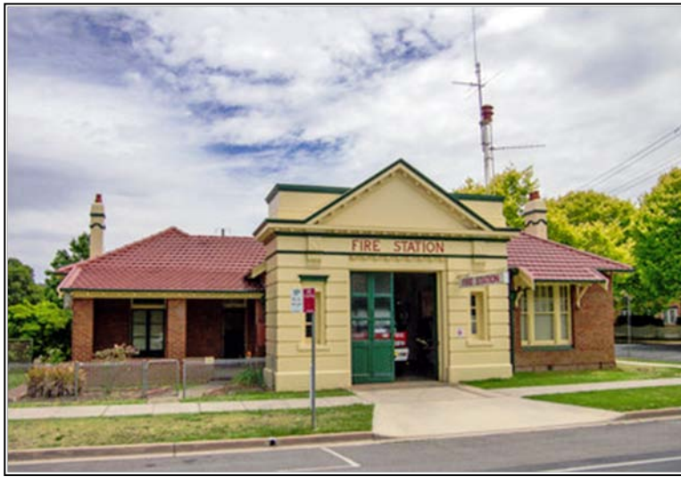
Albury Civic Fire Station
