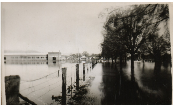
Adelyn factory surrounded by flood waters. The factory itself was not flooded, but the staff had to be ferried to work on the back of a truck.
