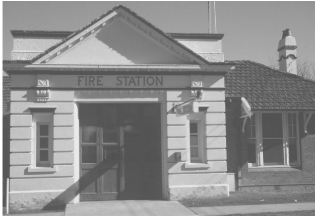
Albury Fire Station Kiewa Street opened in 1916. It was decommissioned in 1980 but recommissioned again in 1983 as Albury Civic Fire Station.
